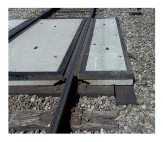
At the locations listed below, the Contractor shall remove the asphalt adjacent to the crossing, remove the crossing panels, replace the existing ties with ten-foot ties, and replace and secure the concrete panels and replace the adjacent asphalt.
