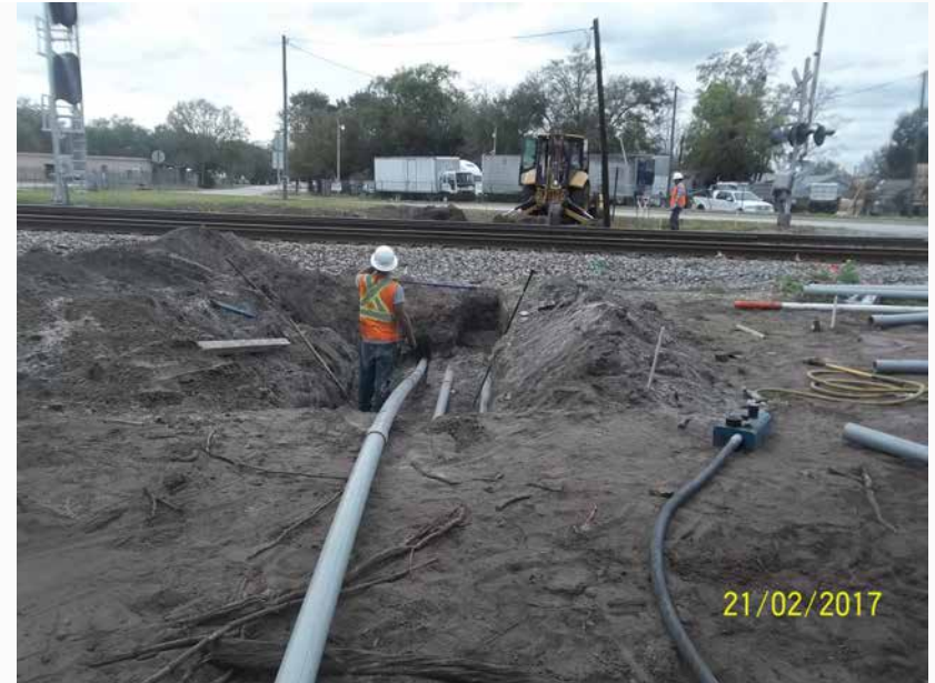
Signal Cable installation btw Pine Street and 4 th Street
