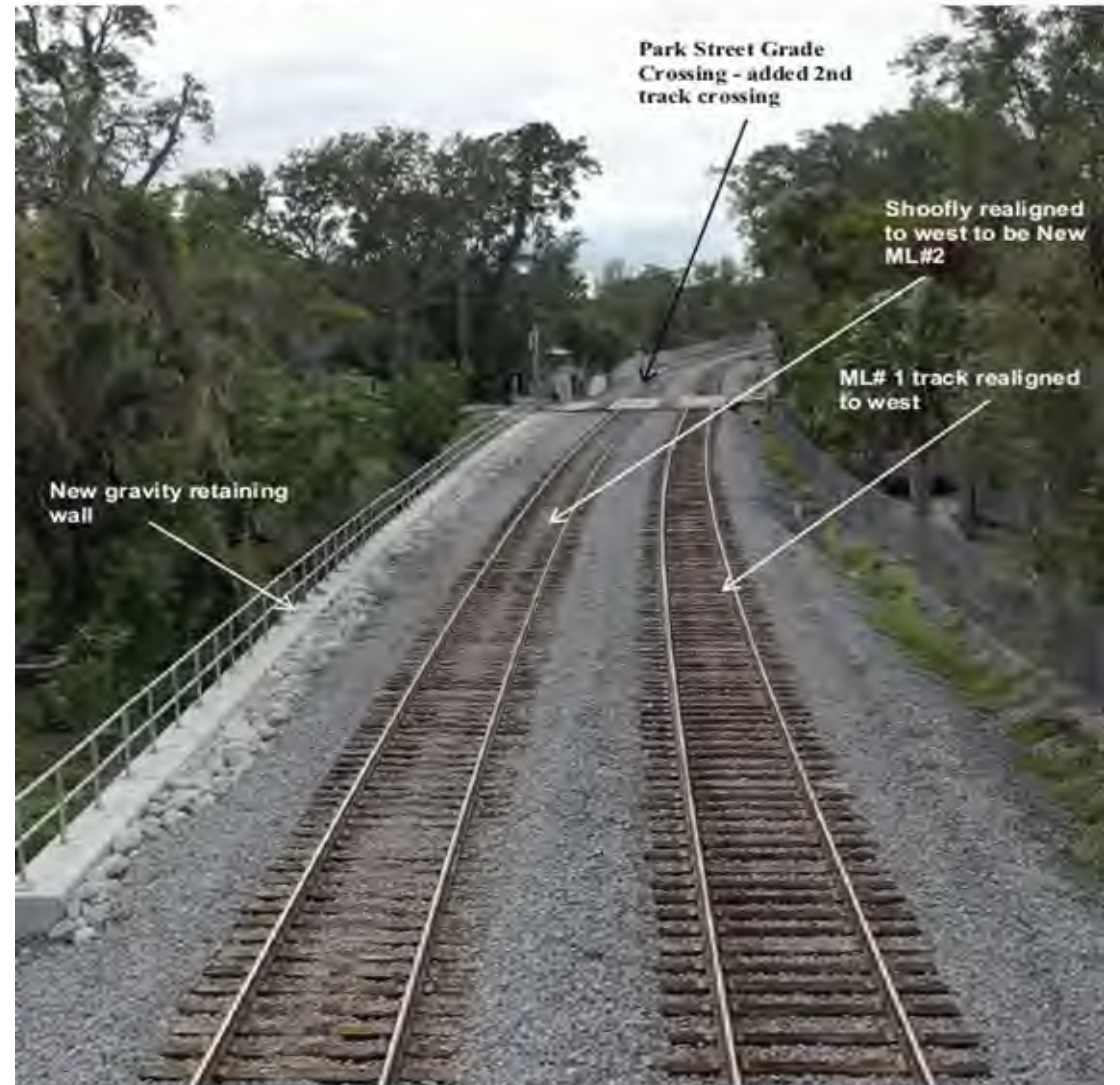
Looking South at Park Street
